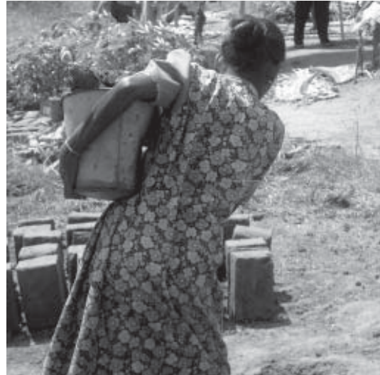
Employing Women: The community contribute by making bricks for their shelters at Pallaiketheikulam
