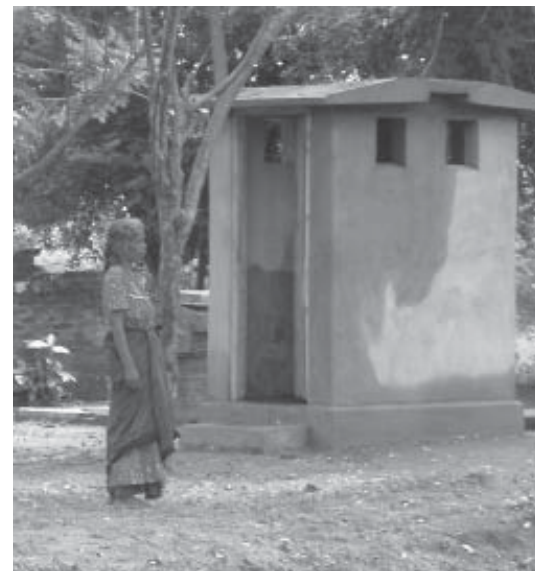
The UNHCR/SLF partnership: providing much needed sanitation facilities in the North.
