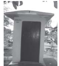
Above > Sewalanka worked with the community to construct water seal toilets.
